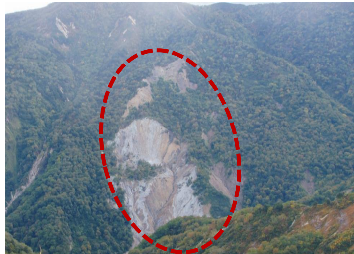
Landslide that occurred in 2015(Forestry Agency)
